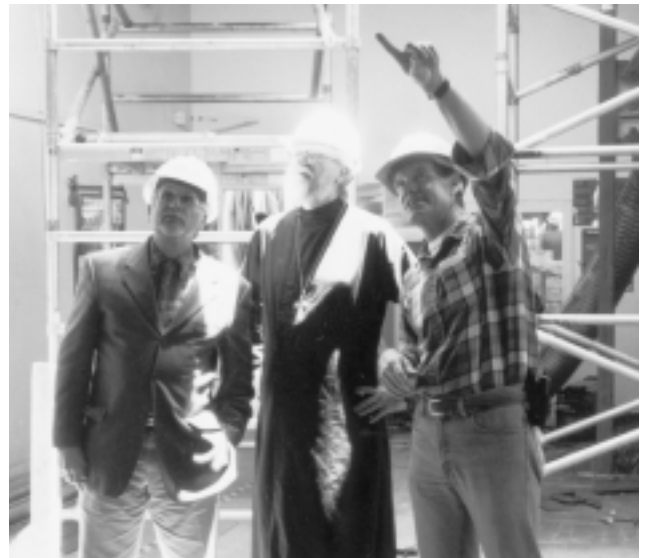
BUILDING FOR THE FUTURE: Surveying the seismic work area (from left): Raphael House board chairman John Hinman, executive director Fr. David Lowell, and DPR Construction superintendent Nelson Vineyard.
